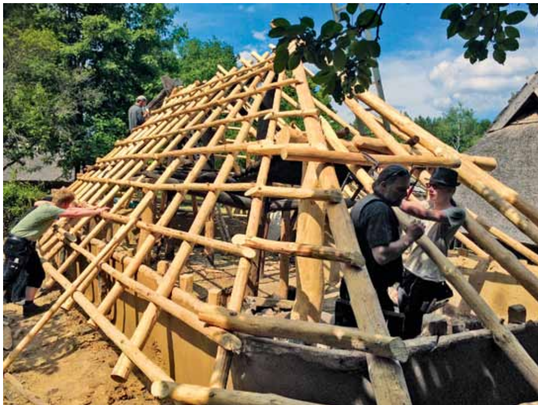
Sanierung eines historischen Hauses. Foto: Julia Heeb Building a new roof for a historic house.
